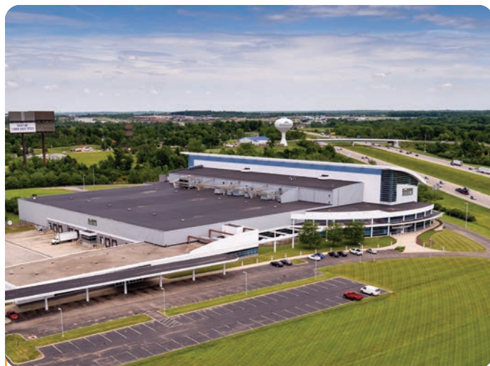
Modula Plant – Franklin, Ohio
