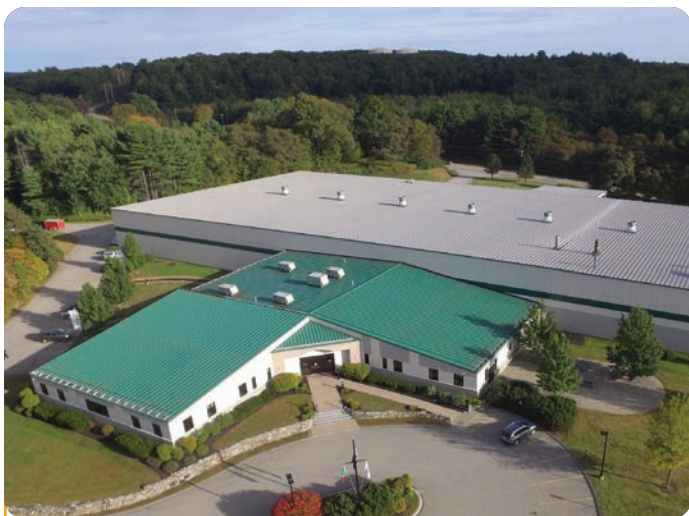
Modula Headquarters and Plant – Lewiston, Maine
